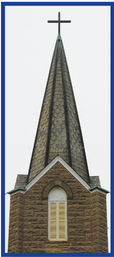
As part of the 1991 Founders Day celebration, a copper cross was installed atop the bell tower.
